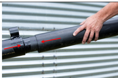
1. Buis verbinding/pipe connection
